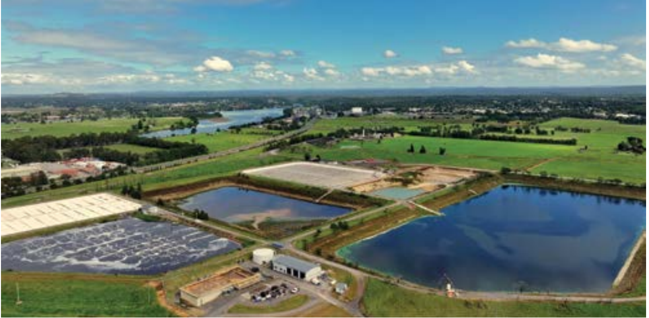
Methane captured from a wastewater treatment facility is used to power the site in Nowra, New South Wales, Australia.
