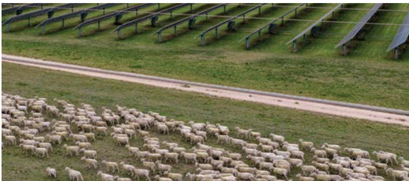
Darlington Point Solar Farm, NSW, Australia.
