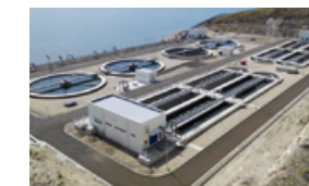
Sewage treatment plant
